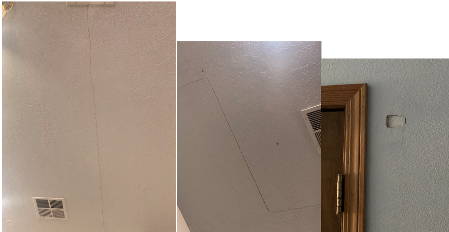
Drywall repairs on our ceilings and various places throughout the building
